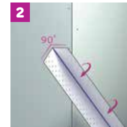
2 Fold the tape along the perforation at 90° or at another°, as the case may be
