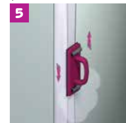
5 Apply a thin layer of jointing plaster to the top of the tape and wait until it is completely dry, sand the dry surface using a sandpaper with min. 200
